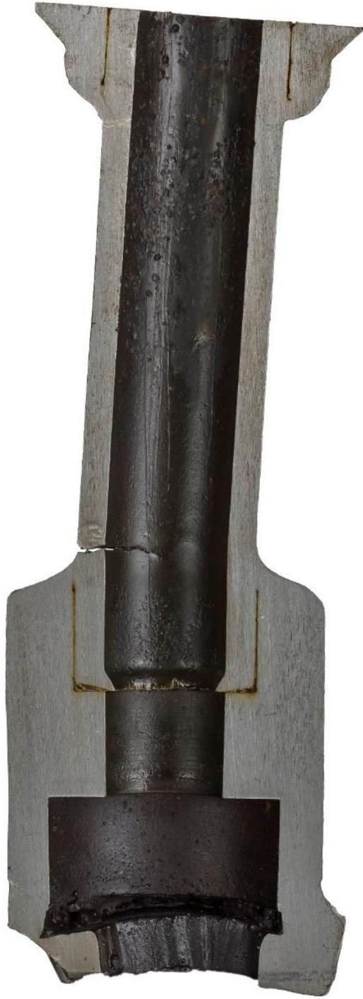
Fatigue fracture of a PI nozzle © CEphoto, Uwe Aranas
