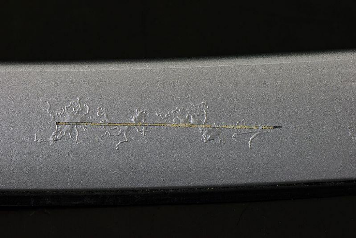
Filiform corrosion spreading from scribe on painted aluminum after complete accelerated corrosion testing (ACT version 2) CC by Matador
