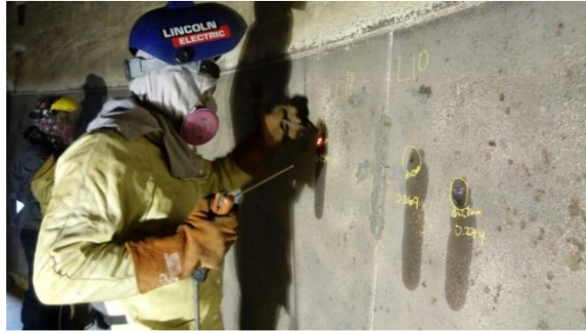
PICTURE 2. FILL-WELDING THIN SPOTS IN THE SHELL.
